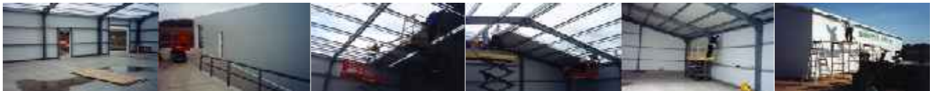
Door openings are cut, framed and capped.
