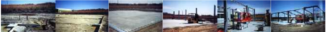
Concrete Piers are aligned and poured in accordance to building specifications.
