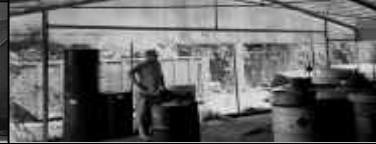
Corrugated Panels Applied on VersaTube Framing (page 73)
