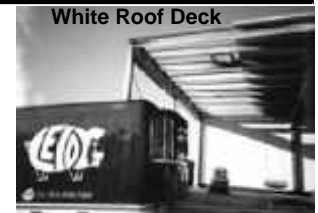
White Roof Deck
